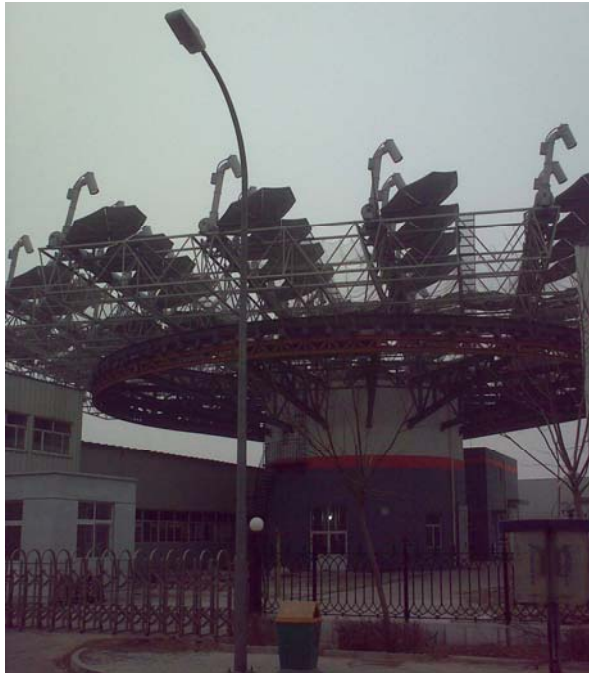
CENICOM prototype, 88 dishes, 150kWp, Tianjin, 2009
