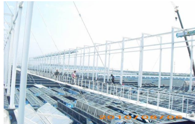
2.5MW Fresnel system under construction, Himin Solar, Dezhou, 2010
