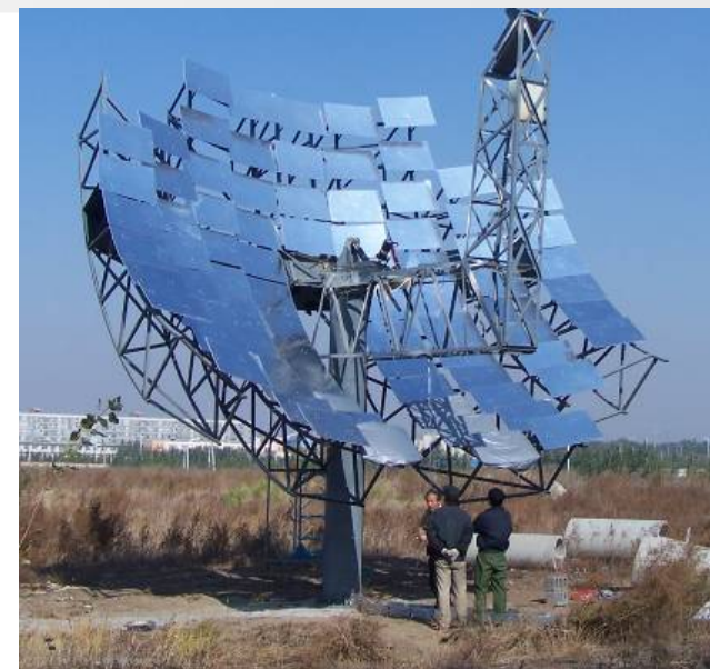
5kW Dish/Thermal Sonic Stirling, technical institute of physics and chemistry, 2009
